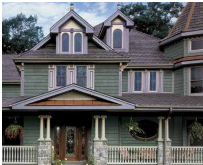
Custom-painted Restoration Millwork
