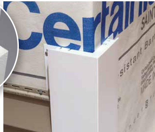
One-piece, smooth 6 in. corner with J-pocket, using InvisiPro flange installation.
