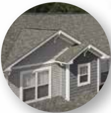
Roofing and Ventilation
