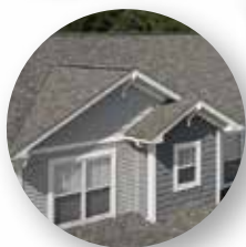
Roofing and Ventilation
