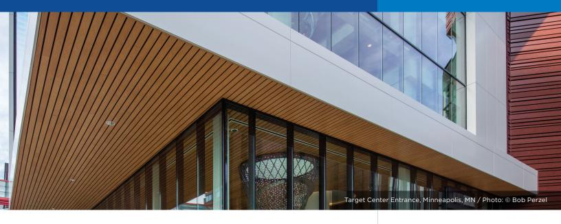
Designed to withstand wind loads, the Deep Box Linear metal ceiling system uses a universal carrier for design and install simplicity.
