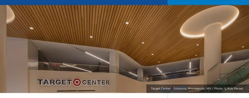
The Deep Box Series linear metal ceiling system uses a universal carrier for simple design and installation.
