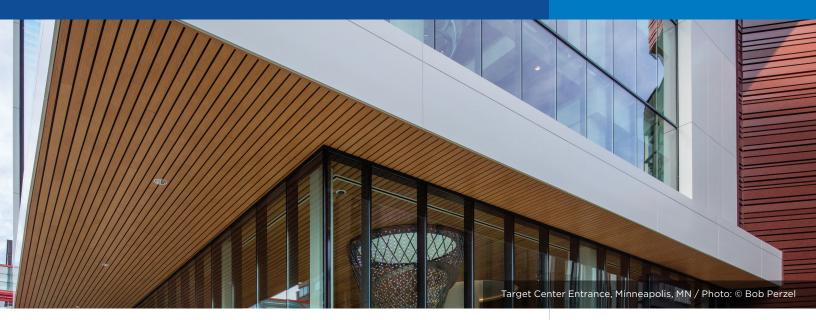
Designed to withstand wind loads, the Deep Box Linear metal ceiling system uses a universal carrier for design and install simplicity.
