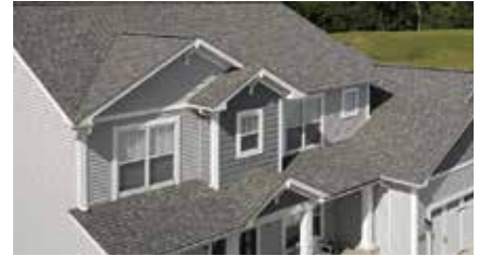
ROOFING AND VENTILATION
