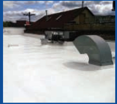
Liquid-Applied Roofing
