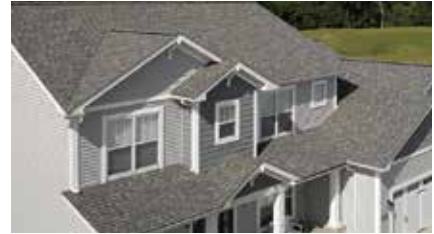
ROOFING AND VENTILATION
