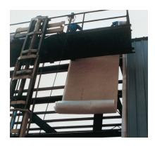
**Benefits:** Metal Building Insulation 202-96 reduces transmission of exterior sound to the interior of the building and absorbs reverberating sounds within the building.
