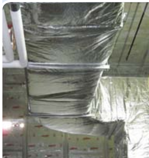
HVAC system installation at the JW Marriot Indianapolis Hotel
