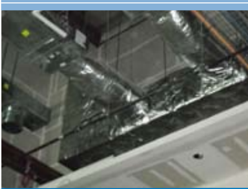
HVAC system installation at the JW Marriot Indianapolis Hotel
