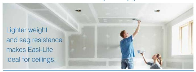
Easi-Lite® can be used on walls and ceilings. For ceiling applications when joists/trusses are spaced up to 24" (610 mm) o.c. the board is to be installed perpendicular. The application of water-based texture is permitted.
