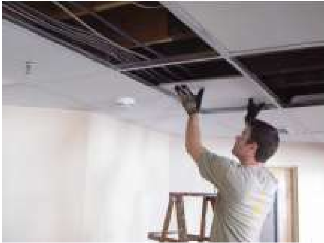
Figure 1: Example Ceiling Panel Installation
