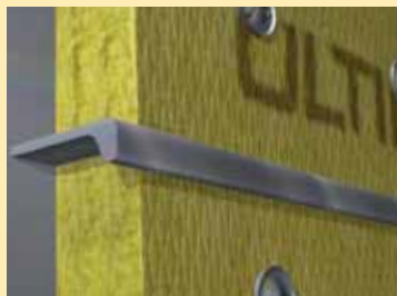
U MPN 24 (24 kg/m 3 ), 100 mm without stiffener insulation
