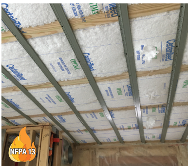
Meets NFPA 13 standard for sprinkler substitution
