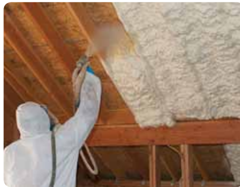
Spray Foam Insulation
