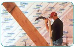
Benefits: OPTIMA fabric is designed to support blow-in closed cavity loose fill installation. During Installation, fabric maintains shape and allows material to flow freely and evenly into the cavity space.
