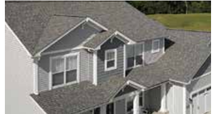
ROOFING AND VENTILATION
