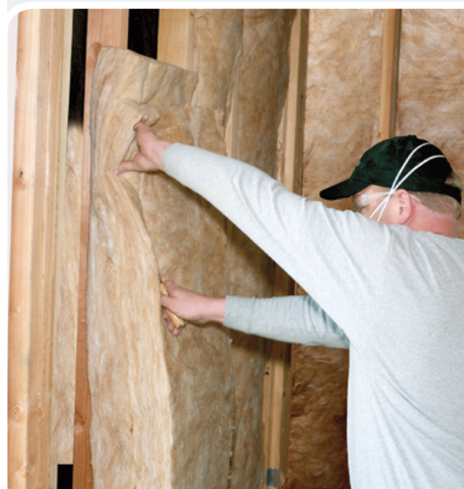
Fiber glass insulation is an effective weapon against moisture and mold damage.
