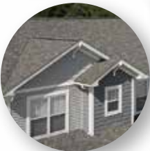
Roofing and Ventilation
