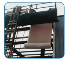
**Benefits:** Canadian Metal Building Insulation reduces the level of exterior and interior noise by reducing transmission of exterior sound to the interior of the building and absorbing reverberating
